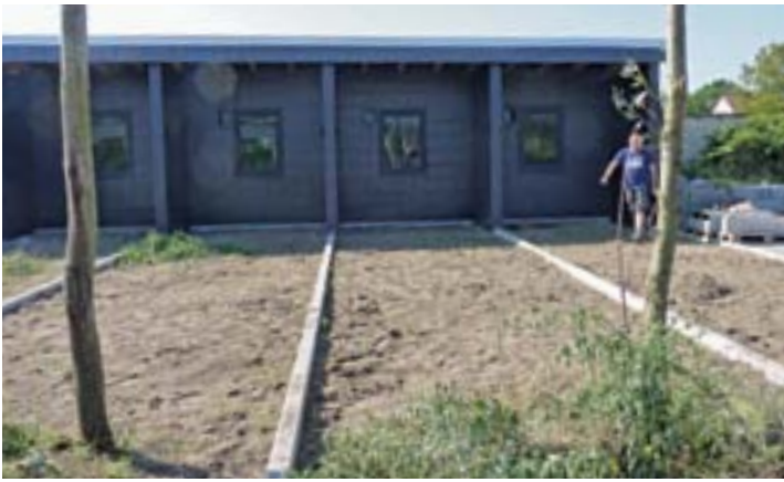
During our visit new aviaries were under construction.
