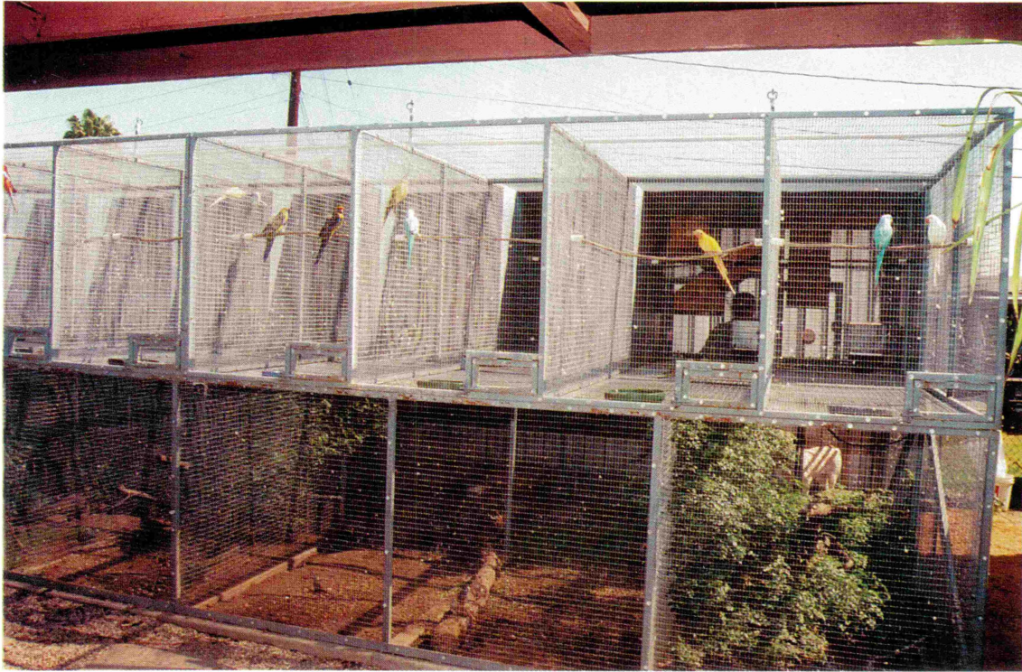
This bank of flights is built on the double-decker plan wherein the upper cages have a floor which serves as a ceiling for the lower cages. The lower cages contain ground birds such as pheasants, partridges, and some ground doves. They can still fly up a few feet to low branches. The upper deck is home to assorted parrots who like to be as high as possible. The dividing bird keeps the birds from bothering each other.
