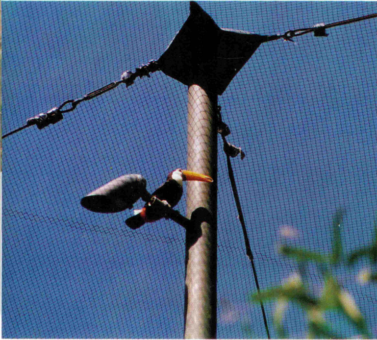
This detail shot shows a huge pole and cables that support the nylon mesh roof of the Leonards' aviary which covers over half an acre.
