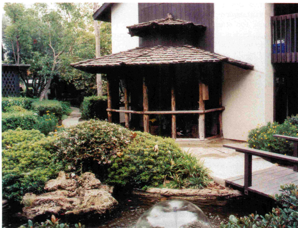
Moss Creek Apartments, Garden Grove, CA. This six-sided unit uses the wall for its backside. It is 12 years old, wood log vertical supports, cedar shake roof and 1/2 x 1/2" wire. The floor is cement covered with redwood bark chips. This apartment complex does live up to its name. It has nice landscaping complete with a fountain and creek.
