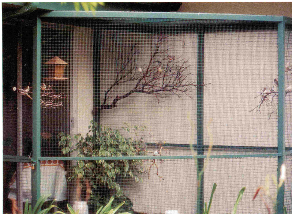
Ashton Court Assisted Living , Orange, CA. This triangular aviary was made to fit in the corner. It is made with 2" x 2" and 1" x 1" steel welded frame with 1 x 1/2" 16 gauge wire. The floor is cement with redwood bark covering. It measures approximately 10' across the front viewing area and 6 1/2' high. It can also be viewed from the window inside.
