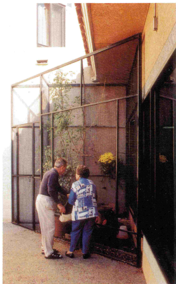
Ashton Court Assisted Living , Orange, CA. This triangular aviary was made to fit in the corner. It is made with 2" x 2" and 1" x 1" steel welded frame with 1 x 1/2" 16 gauge wire. The floor is cement with redwood bark covering. It measures approximately 10' across the front viewing area and 6 1/2' high. It can also be viewed from the window inside.
