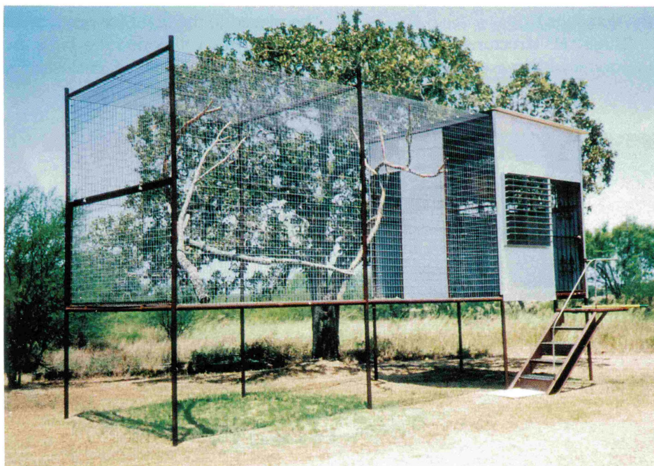
Open all Summer. The hinged winterizing panel is swung to overlap the center portion of the interface. The sliding access door is fully opened between the interior cage and the open flight. The vent on the east side is fully open and the flexiglass panel has been removed from the keeper's entrance door.
