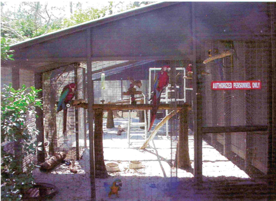
An attached flight made of aluminum construction. The frame was built by a screen enclosure company. They added aluminum panels at the top that function as perfect windbreakers where the sleeping perched are placed. Floor is wired then covered with sand that rakes clean easily. There is an identical entrance a both ends of the aviary. Perches are made from dead cypress trees and are replaced about once a month. Natural foliage protects and beautifies the outside. A section of roof is covered, the rest is open.
