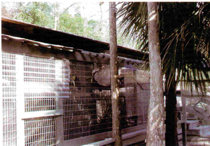
This 40 x 16 foot long aviary houses toucans. It lines up against the house. Low door enters to an inner space with a secondary door to the bird enclosure. Two types of plastic panel are used as weather protection, inexpensive panel for top and heavier acrylic bung with S books for removable side protection.
