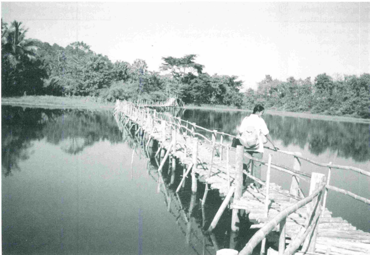
Once in the bird sanctuary there are islands amidst the waters. This bamboo bridge called “Watcher’s Walk” was contributed by numerous bird watchers to make this part of the sanctuary accessible to visitors even though it is across a stretch of water.
