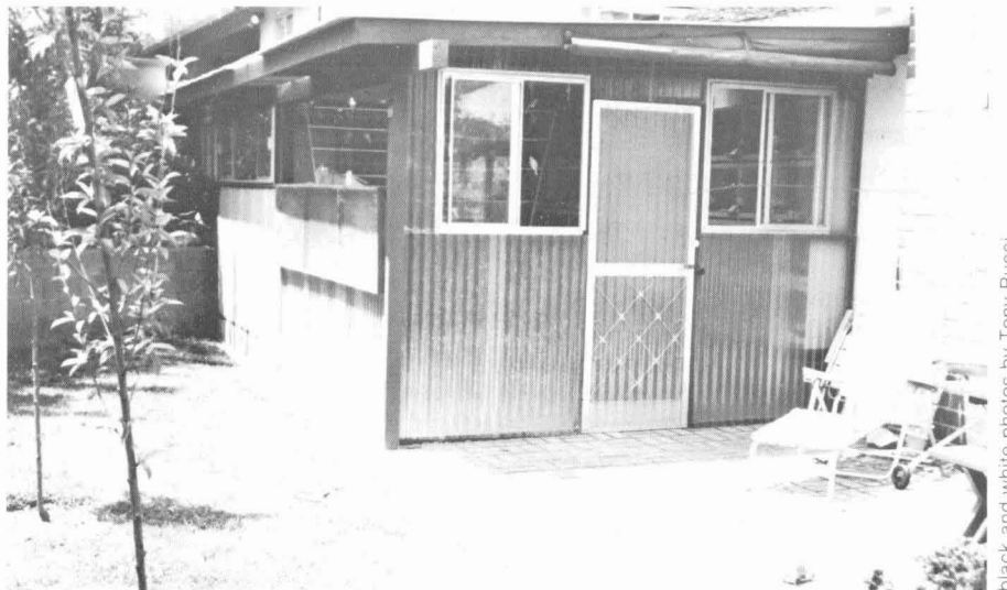
The Bucci's enclosed patio serves as a bird room.
