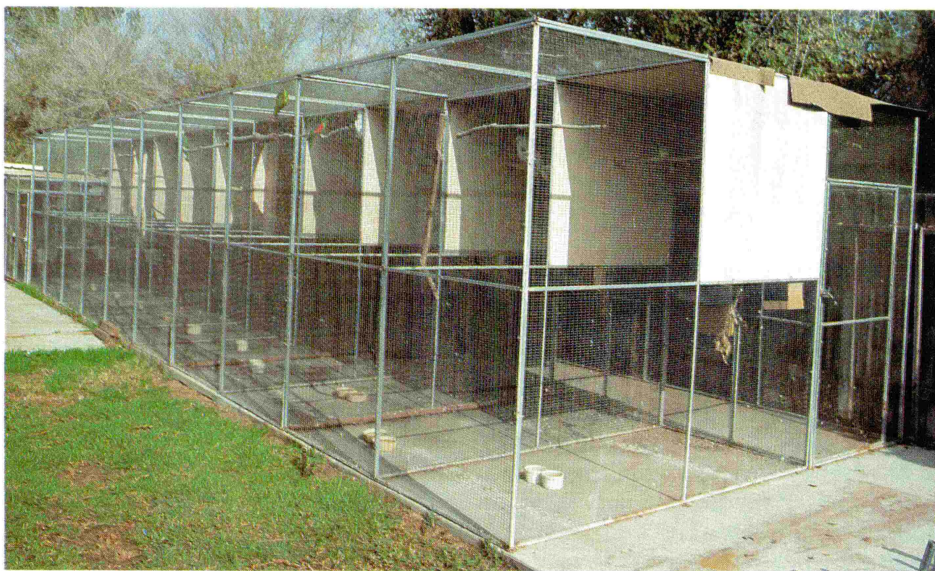
These 4' x 8' aviaries are ideal for medium sized parrots. The safety zone to the rear provides access to the flights for feeding and checking nest boxes. There are 1/4" spacers between the steel frames and concrete floor to allow easy drainage.
