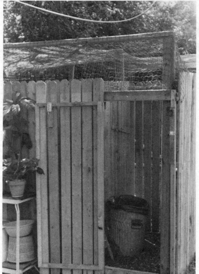
An entrance hallway is necessary to prevent escapes and provides a useful area for the storage of maintenance supplies.
