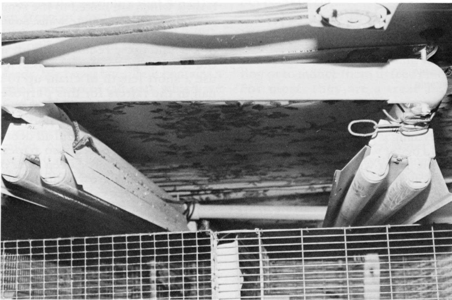
PVC pipe light stands are designed to provide proper lighting to each cage.
