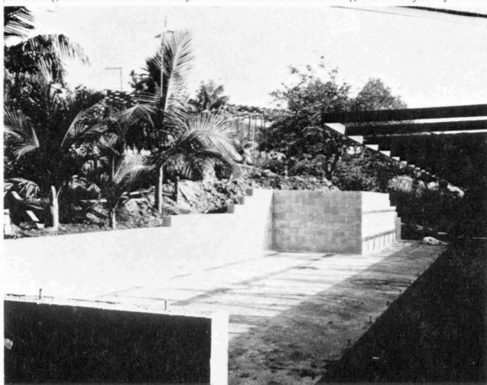
Looking north, view shows finished slab and retaining walls before framing.
