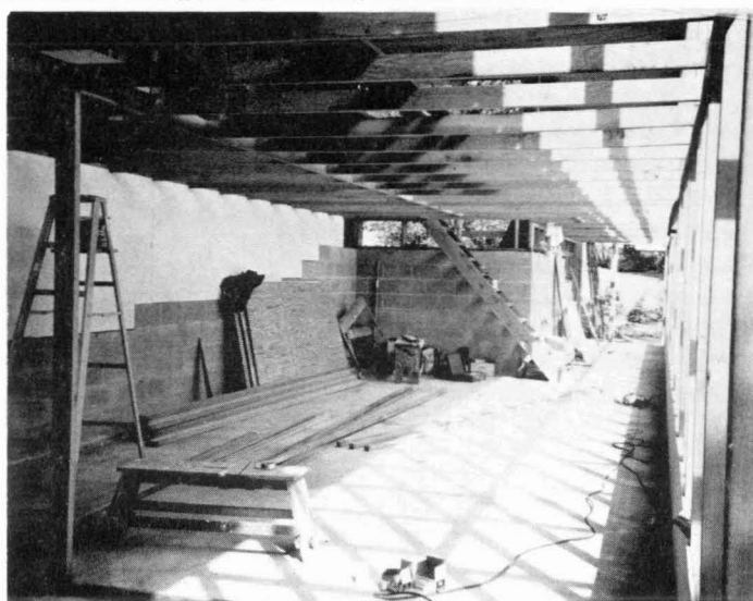
Downstairs during framing showing staircase center rear.
