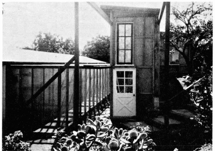
Same view showing entrance after framing.
