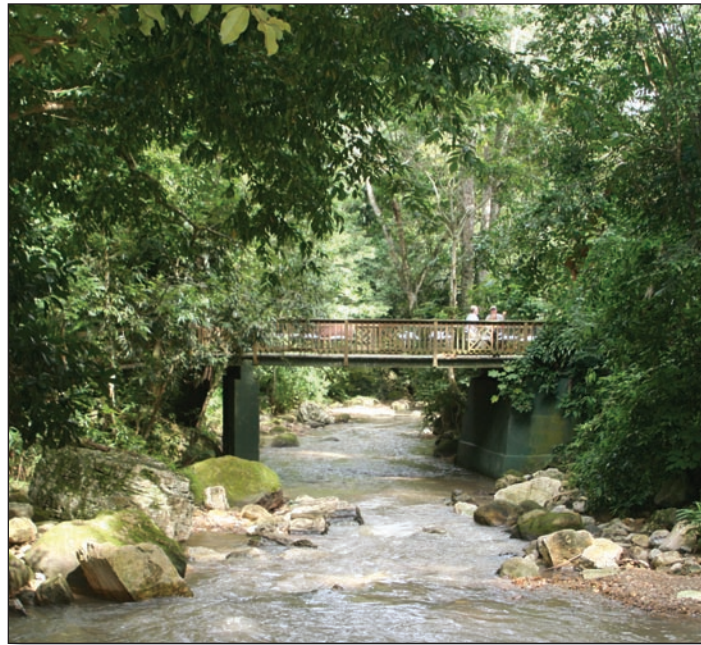
The large bridge over the river doubles as the outside eating area of the restaurant.
