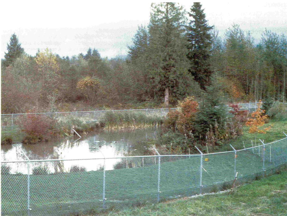
Predator-proof security fencing. Note electric fence wire eighteen inches above ground.
