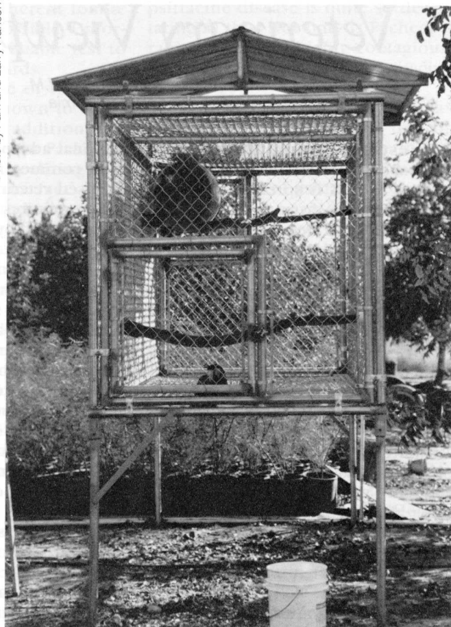
Macaw cage is 14' long, 5' high, 5' long and raised 2-1/2 feet off the ground by its metal post framework. Roof covers back half of cage. 30 gallon plastic drum nestbox has a rear inspection door.
