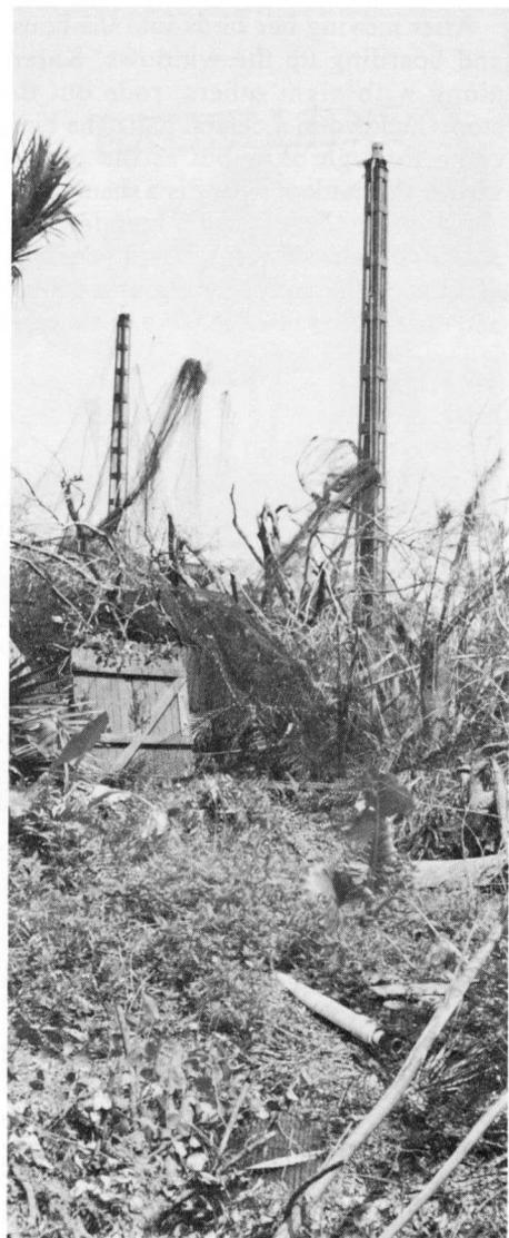
*The remains of Wings of Asia . . . heavy aviary netting was torn and wadded up like thin gauze, clumps are left hanging from cables supported by these towers. Instruments on site recorded winds at 165 m.p.h. with gusts to 200 m.p.h.!*
